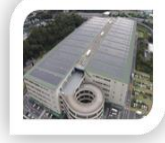
Location: NagareYama Size: 2.3MW
