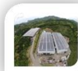
Location: Nagasaki Size: 2MW
